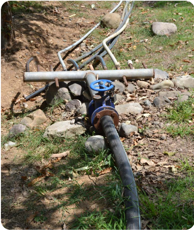
Top: Inside the 240,000-litre concrete reservoir. Bottom: Distributor of water from the main plastic pipe to the valves at the plots ©Sustainable Caucasus
