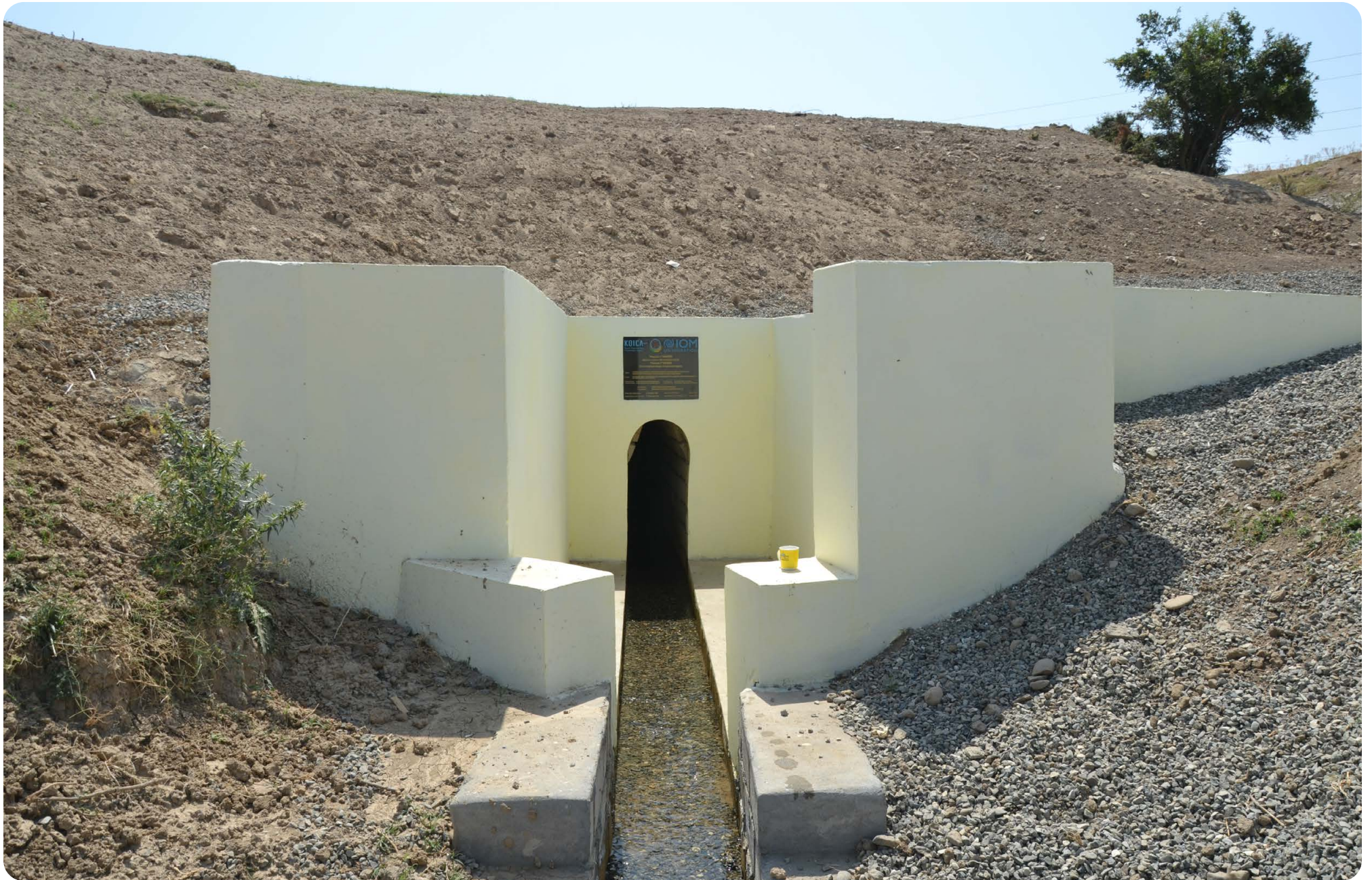
A rehabilitated Khariz providing water in Agdam district, Azerbaijan ©Sustainable Caucasus
