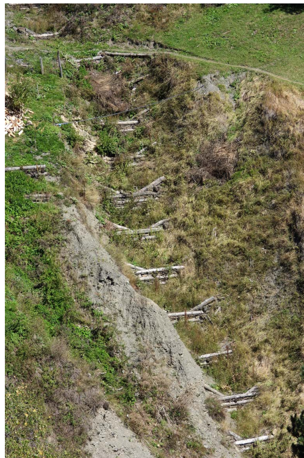
Left: Sketch of the structure of wooden check dams (from Rauch, Rauch and Kirchmeir 2016). Centre and right: Wooden check dams installed in a gully in Jvarboseli village (before and after) ©Deutsche Gesellschaft für Internationale Zusammenarbeit GmbH (GIZ 2019/Sustainable Caucasus)
