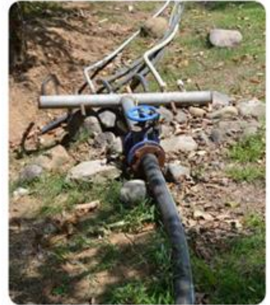
Top: Inside the 240,000-litre concrete reservoir. Bottom:
