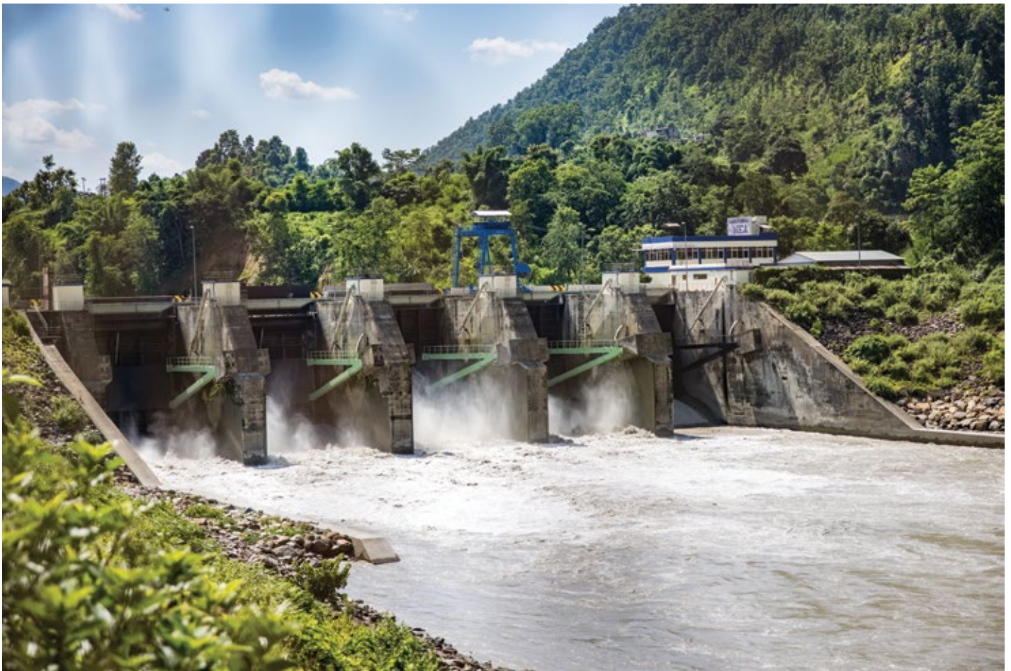
MARSHYANGDI HYDROPOWER PROJECT, NEPAL
